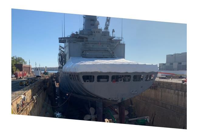
Using cable to create a dome, we then installed the Global Wrap 12 mil, fire retardant shrink film over the ship to create a drum tight, seamless enclosure that prevents dust particles, water and other debris from entering an area being recoated or painted. It also enables work to proceed when it rains or snows.
