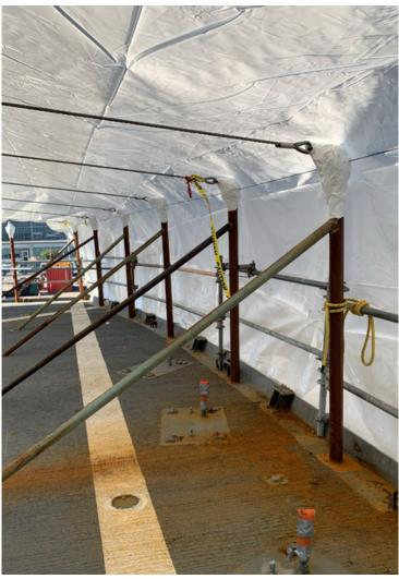
Many projects call for designing a support system using aircraft cable as shown in the images of our most recent installation. In order to support the film dome, the cables are installed at 8 – 10ft at the center and are attached to the vertical stanchions. They are then welded into place around the perimeter of the flight deck to keep the dome up 6ft from the deck. There are also attachment points on the main housing of the superstructure.
