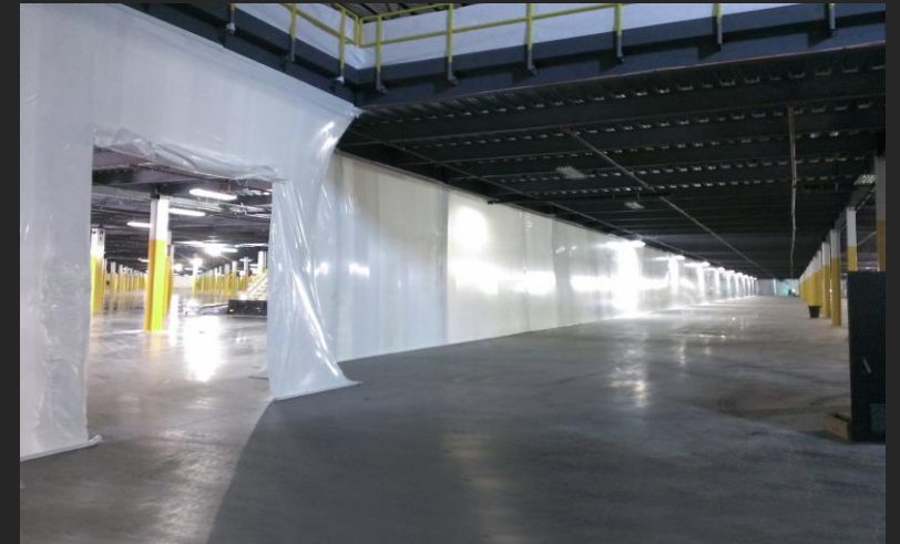
Temporary Dust Barrier Walls
